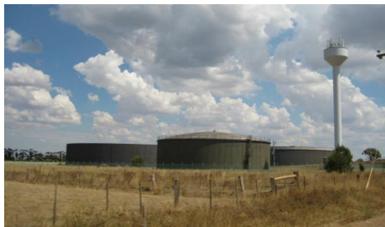
example of major infrastructure within the green wedge
